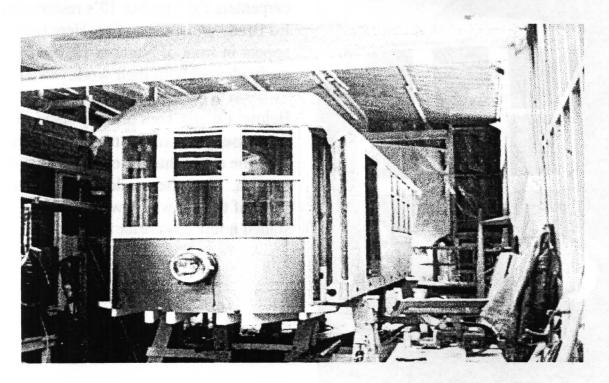
Above: Number 10 with north vestibule rebuilt, a new roof and siding and windows installed awaits the delivery of its trucks.
