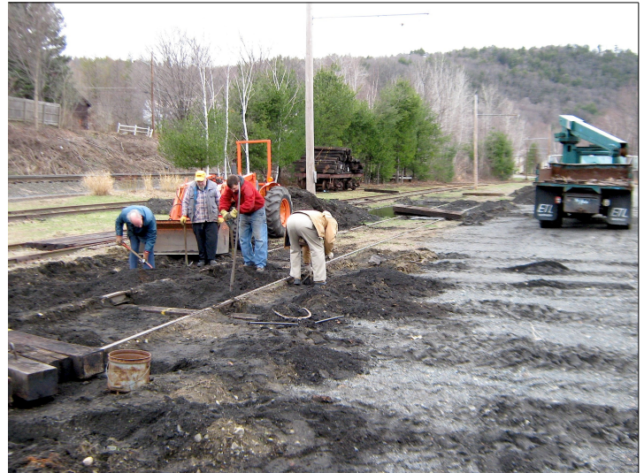
Trackwork is already in progress at SFTM. Under the supervision of John Greene, Dave Goff, Bill Kaiser and Bill Townsend put muscle to coaxing yet another replacement tie into place.
