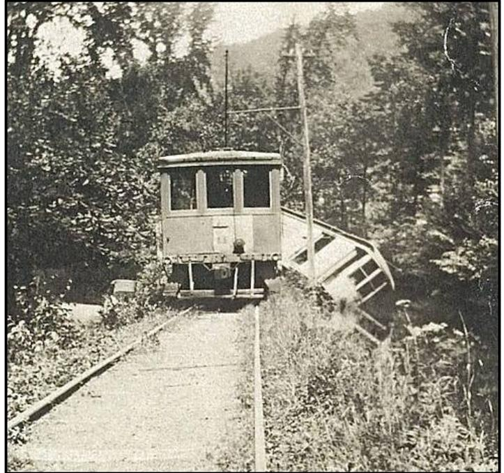
Car No. 25 to the rescue. 25, like 10, was a combine, but it was built to handle interchange cars with the B&M at Shelburne Falls. Note railroad coupler, air hose, and poling pockets.
