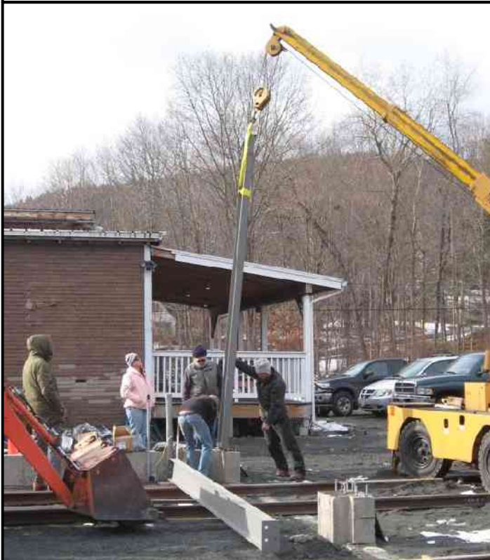
The anchor bolts really do line up. Lucky so far. But just wait!!
