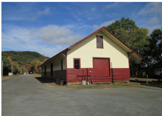
Exterior Restoration of the Freight House is complete!
