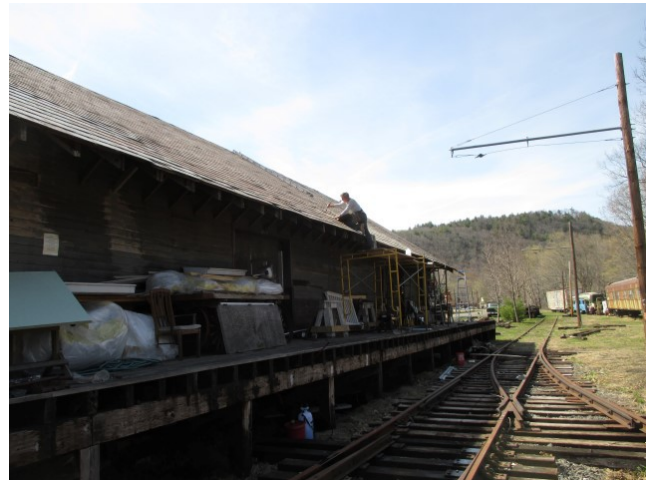
Jerry adds slates where the dormer used to be.
