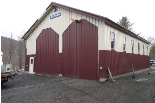
The west end of the new Car barn.
