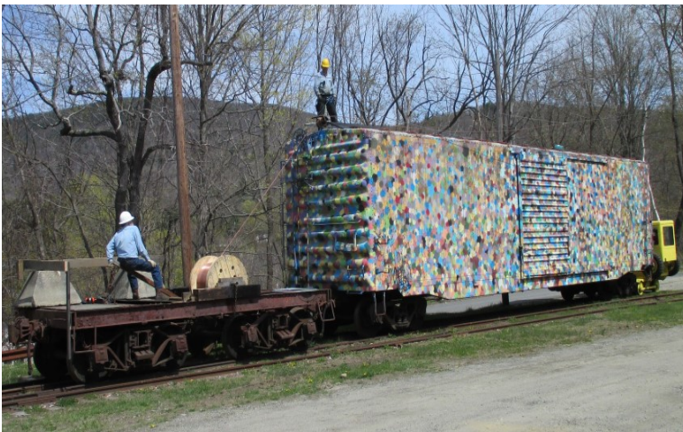
The "Wire Train" hangs the new trolley wire.
