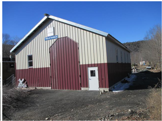
The east end of the new Car barn.
