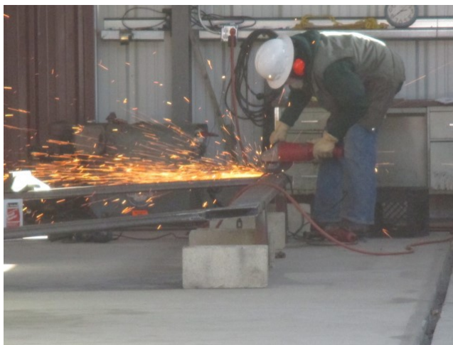
Larry smooths the welds on a door frame.
