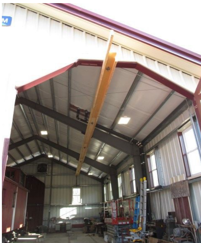
The overhead trough for carrying the trolley wire
