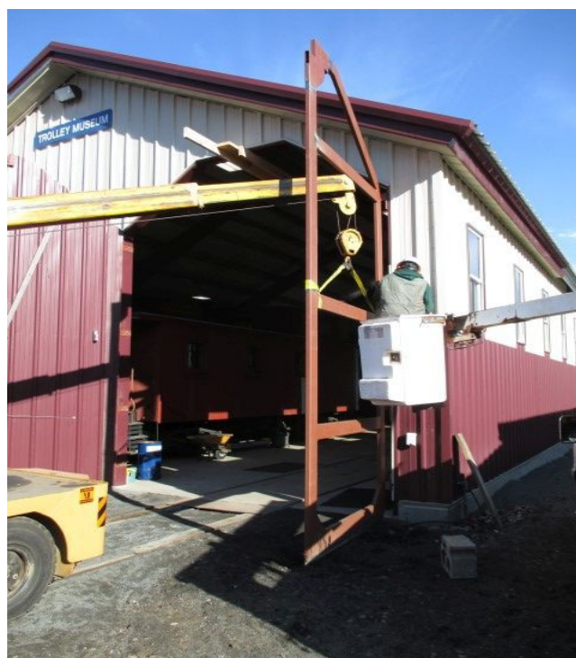
Larry, with the Drott crane and the Bucket Truck, hanging the last door frame
