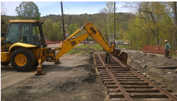
Hillman Bros backhoe tweaks the track alignment.
