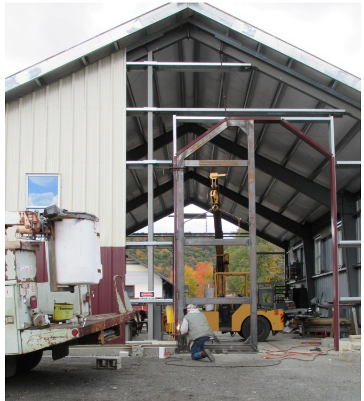
Larry welds hinges on the Car Barn doors.
