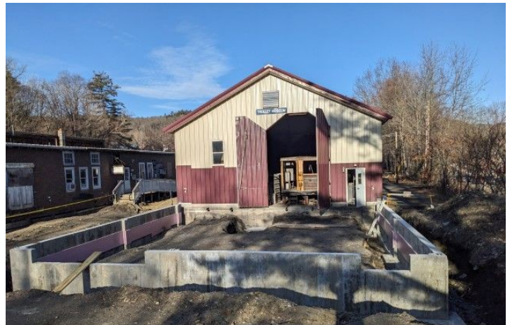
The foundation is poured for the Car Barn Extension
