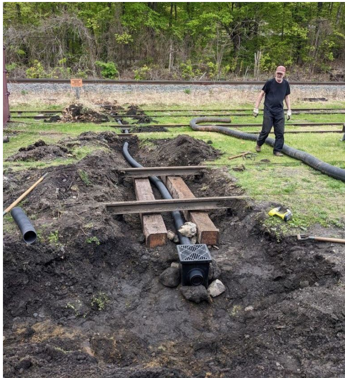
Nash inspects drainage project on Main Track
