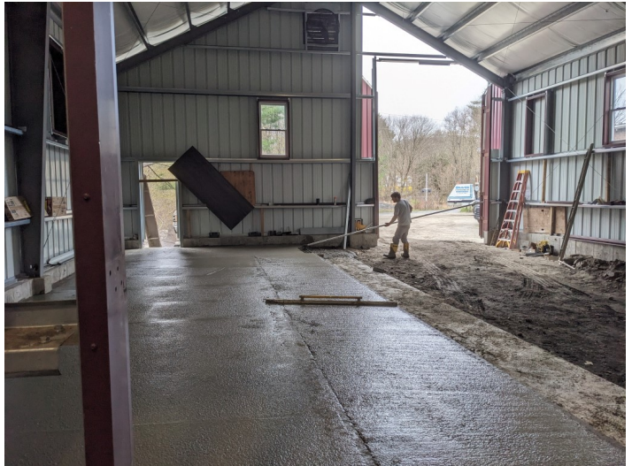
May 2024 - Stall One done, Stall Two being prepared
