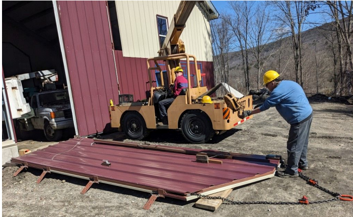
April 2024 - Martin and Nash install a door panel
