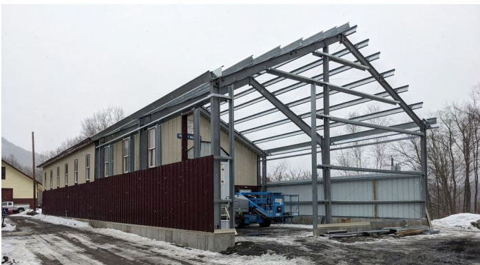
Jan 2024 - All the framing and some siding is up
