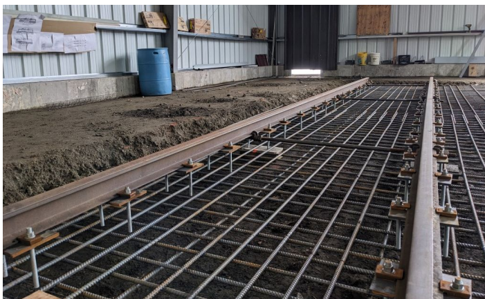
April 2024 - Stall One ready for sub-floor pouring
