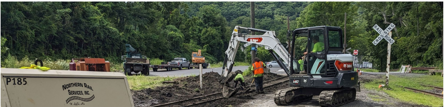
Above - Northern Rail Services replaces ties in our Main Track. Below- Martin keeps No. 10 looking spiffy and Tom builds some new pieces for the "Berkshire Hills" trucks.
