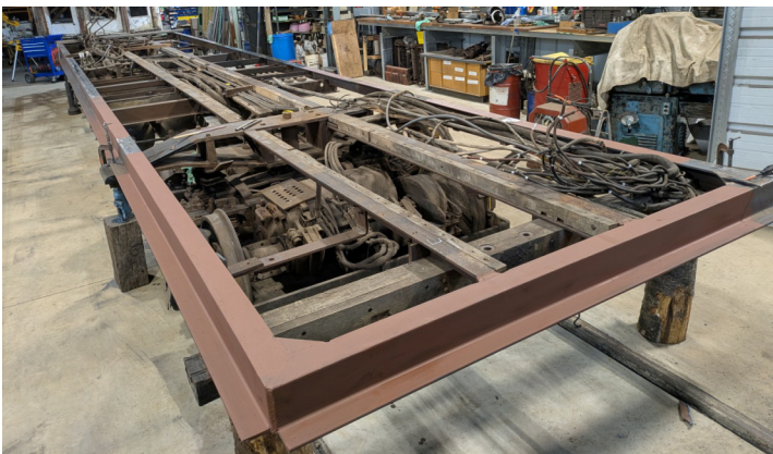
The rotted parts of the underframe have been completely replaced and partly primed
