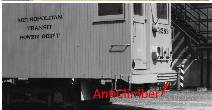
Upper: New bumpers with anti-climbers Lower: Showing anti-climber as delivered, Kevin Farrell collection
