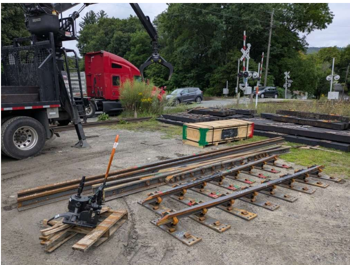
Switchstand, frog, points and timbers awaiting installation by Berkshire & Eastern Railroad
