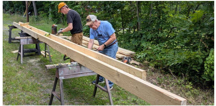
Nash and Phil build the wooden trough for the trolley wire in Stall One, upside down for easier assembly.
